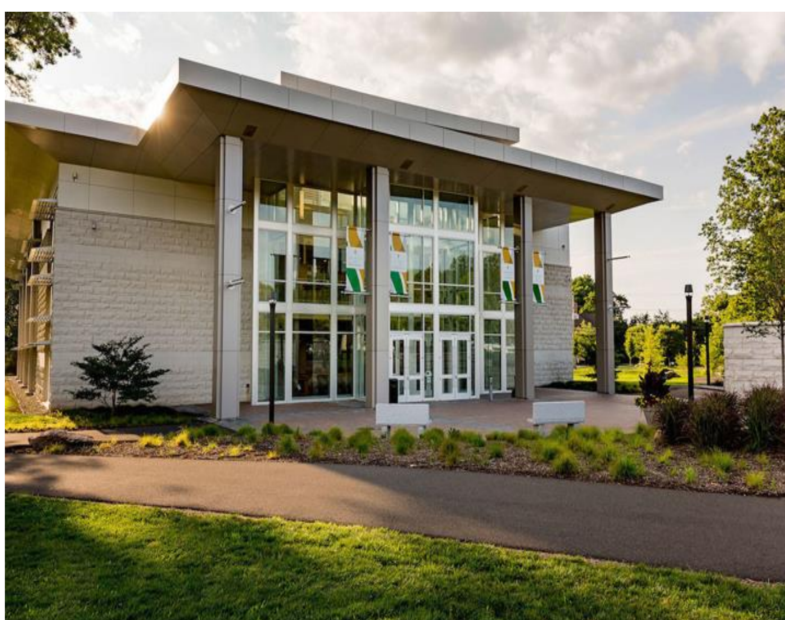
Figure 1. Life Sciences Building (LSB) of Delaware Valley University.
